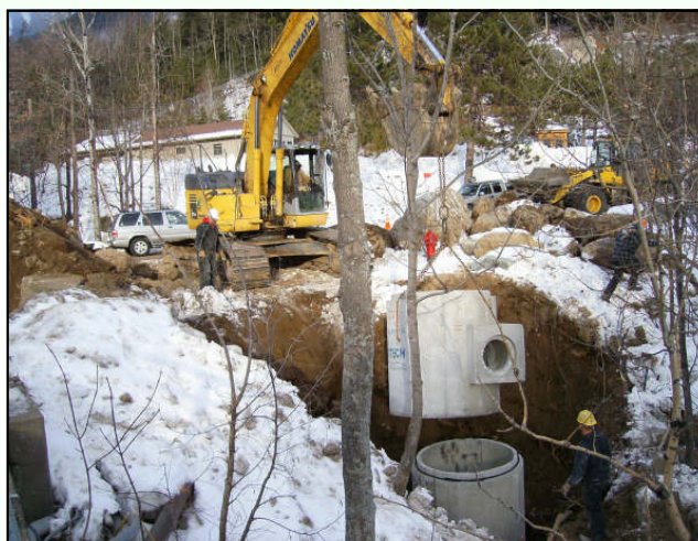
Construction of Vortex Filtration Unit at Whiteface Mountain (above)
