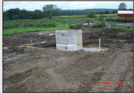
Installation of Milk Center Wastewater Collection (Washington County)
