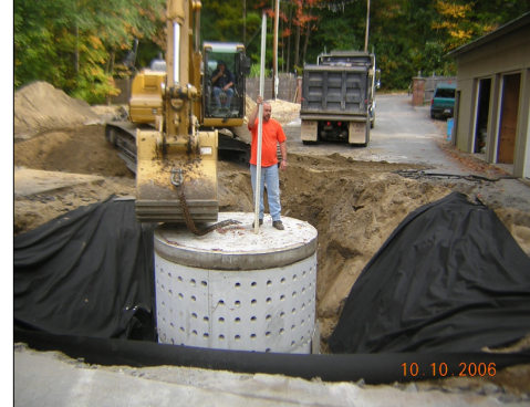
Installation of Stormwater Filtration System in Prospect Mountain Brook Watershed, Lake
