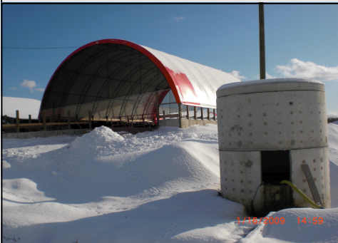
Milk Center Wastewater system installed (Washington County)
