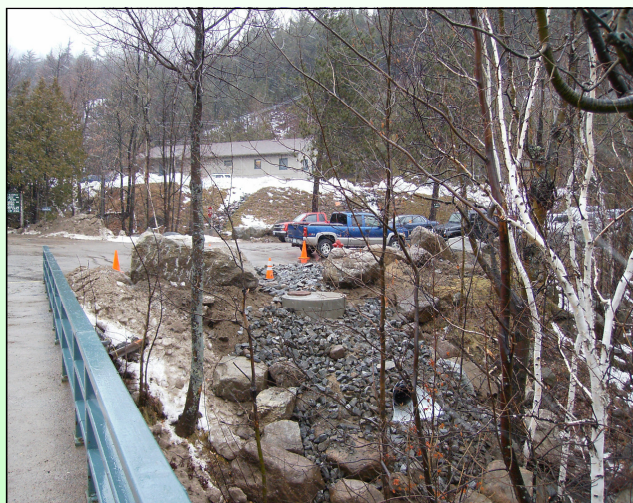
Vortex Unit Installed at Whiteface Mountain
