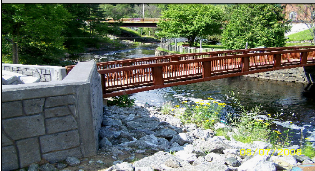
Post Construction Stabilization and Sediment Containment. River Walk, Saranac Lake.
